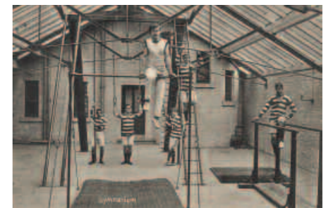
A very early 'Sports Hall' circa 1910 (now the boiler room).
